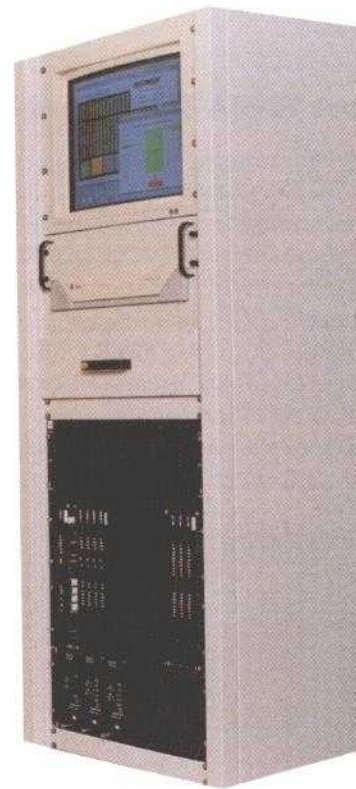
COMSAT Laboratories' high-data-rate gateway switch is installed at the Southbury and Santa Paula land earth stations.
